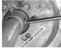
reinstall stopper screw and tighten set screw
