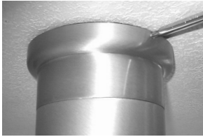
secure with set screws
