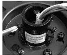
loosen screws on coupler
