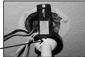
(12) With fan safely suspended by bracket, make wire connections with wire nuts included in hardware package as described in the **Control Installation Instructions**. If using optional #003, #004 or #005 controls, the receiving unit should be placed inside the arms of the hanging bracket and connected at this time.
