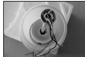
(11) Lift fan to ceiling and set half ball in the hanging bracket so that the ridge on the edge of the hanging bracket is seated in the slotted channel in the half ball.
