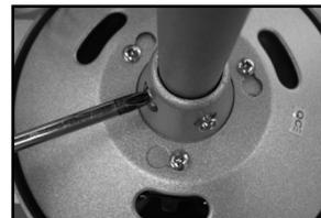
(8) Slide fan canopy over down rod and carefully rest on top of fan body.
