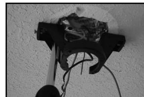
(3) Remove top cover by loosening the three screws holding it in place. Set cover aside to replace after blade installation.
