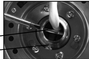
**(8)** Run fan wires through selected down rod. Reinstall stopper screw from step **(7)** and firmly tighten set screw on fan collar against down rod.
