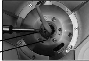
(5) Run fan wires through selected down rod. Reinstall stopper screw from step (4) and firmly tighten set screw on fan collar against down rod.
