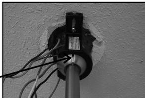
(10) With fan safely suspended by bracket, make wire connections with wire nuts included in hardware package as described in the **Control Installation Instructions**. If using optional #003, #004 or #005 controls, the receiving unit should be placed inside the arms of the hanging bracket and connected at this time.
