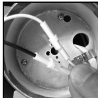
**(b)** Attach socket and bracket to fan using screws from hardware package.
