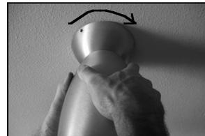
(9) Insert and firmly tighten three canopy screws from hardware package.
