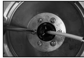
(6) Using security cable and hook, suspend fan from hugger mounting plate. The suspension hook should be inserted through the open hole on the fan motor coupler.
