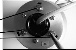
(4) Place hugger canopy on top of fan body so that larger holes fit over small screw heads and smaller holes are aligned with open screw holes from step (3).
