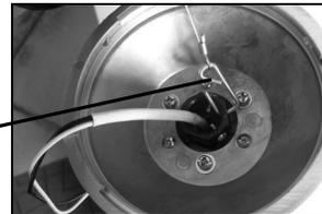
(7) Using wire nuts included in hardware kit, make wire connections to power supply in junction box: black to hot and white to neutral. Excess wire can be trimmed prior to making connections for easier wire management. **CAUTION:** power must be turned off at switch location or at circuit breaker prior to handling wires. DO NOT perform wire connections with live/hot wires.
