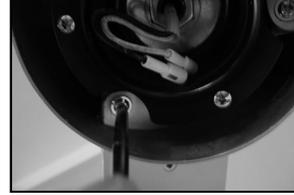
**(24)** Make connections from light socket plate to wire leads coming from the bottom, center of fan body.
