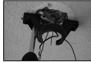
(11) Remove the cotter pin, washer and stopper pin assembly from the small down rod and set aside for step (14).
